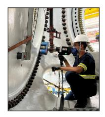
Reliable tools are fundamental for fastening critical bolts in wind tower construction. Particularly in a wind tower hub that must transmit and withstand significant load, it is essential that bolting tools reliably and consistently meet strict tolerances. AcraDyne DC HT Extreme Duty tools not only are able to meet these exacting demands, but also have proven to be exceptionally durable.
